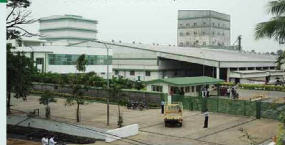
Front and entrance view of Growel Feed plant
